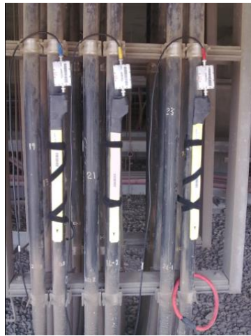
Example of FMC on high voltage cable with IP68 protection cover
